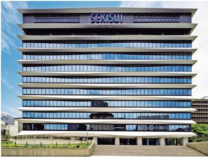
The renovated Osaka Head Office
