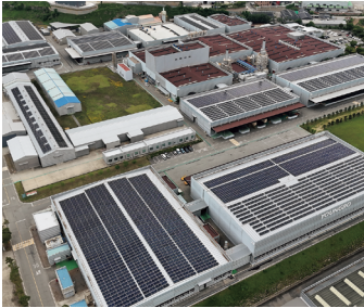
Youngbo Chemical Co., Ltd. Cheongju Plant
