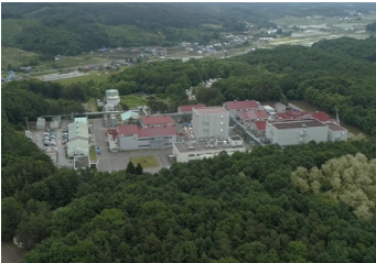
Panoramic view of Iwate Plant
