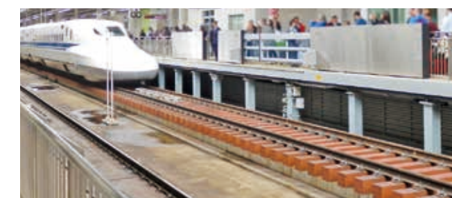
Track built on synthetic railway sleepers for Line No. 27 at Shin-Osaka Station
