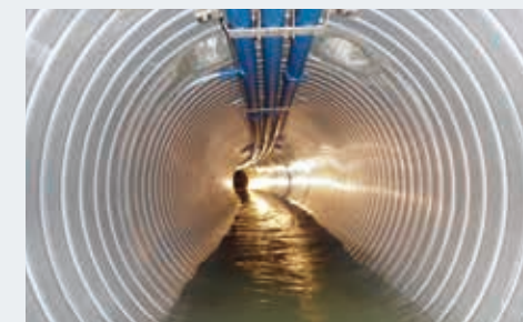
Sewage conduit after Esloheat sewage heat construction work
