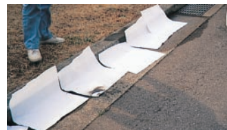
Tsukuba R&D Institute Prevention of outflow of alkaline solution at the time of disposal
