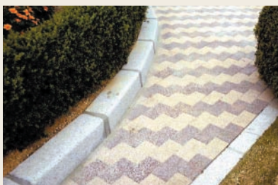
Light-weight water penetration paving blocks (Picture 1)
