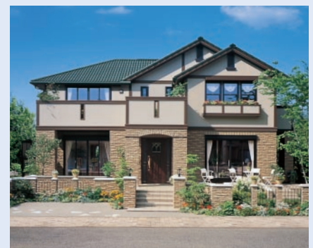
"New Miore" With a Photovoltaic/Thermal Hybrid System and heat retaining flooring
