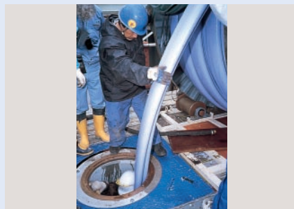
Omega Liner Relining Pipe (Renewal of small diameter sewer lines, resource saving)
