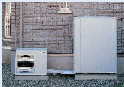
Hot Water Unit with CO 2 Heat Pump (No chlorofluorocarbon media, less emission of carbon dioxide than electric hot water unit or gas hot water unit)
