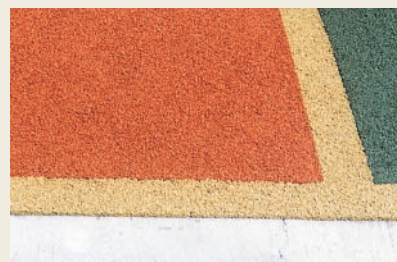
Water penetration resin pavement (Picture 2)
