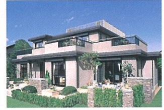
"Sekisui Heim Parfait®" Home equipped with photo-voltaic generation system reducing CO 2 emission by about 2.0 tons a year
