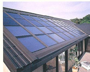
Photo Voltaic-Thermal Hybrid System About 2,300 kWh electric power can be saved a year in a standard home in the Tokyo district
