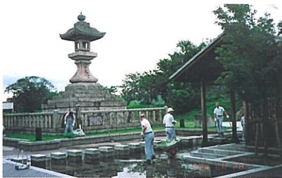
Cleaning all-night lights at Tokaido-Yokota-watashi/Shiga-Minakuchi Plant
