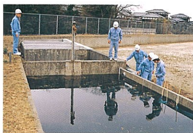
① Outflow prevention by shutter-gate
