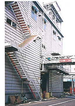
Resin factory extension (Shiga-Minakuchi Plant) Adopting specifications for energy saving such as use of highly efficient motors, rotation control by inverters, etc.
