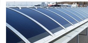
Film-type perovskite solar cells installed at the Gate Transportation Terminal at Expo 2025 Osaka, Kansai, Japan
