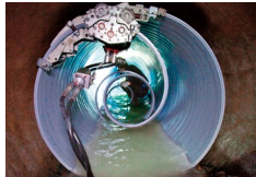
SPR Method contributes to the renewal of aging infrastructure, including sewage pipes
