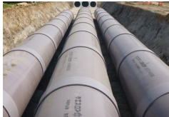
Reinforced plastic composite pipes are also used as rainwater storage pipes
