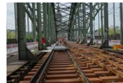
Synthetic sleepers for railroads have exceptional water resistance and durability
