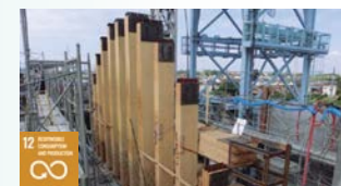
SEW Work Method (Shield Earth Retaining Wall System)
