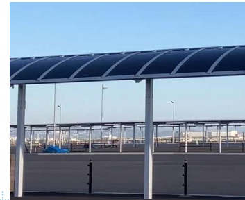
Construction example (Osaka/Kansai Expo)
