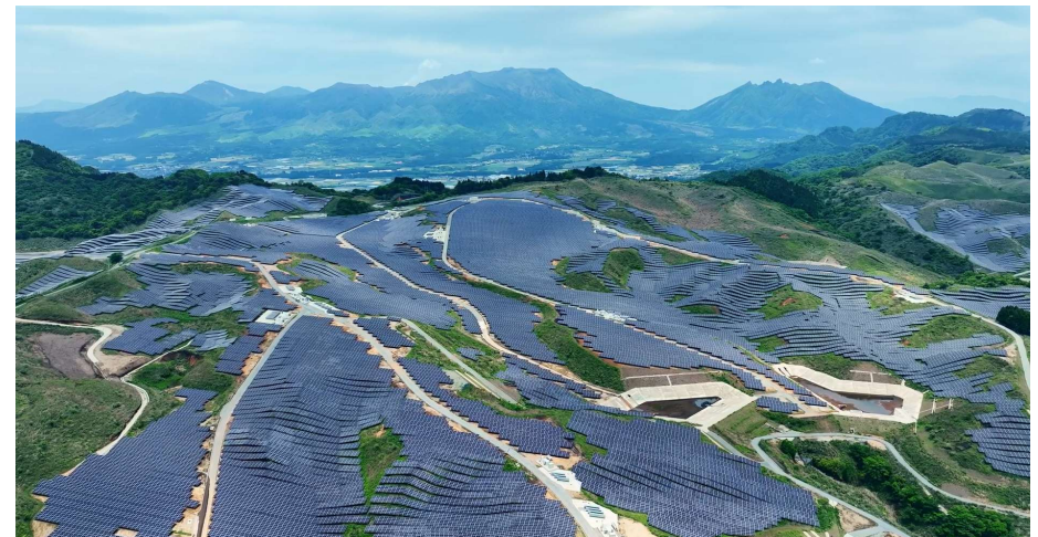
Mega solar panels over the Aso mountains
