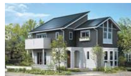
Wooden modular house (SEKISUI Two-U Home)
