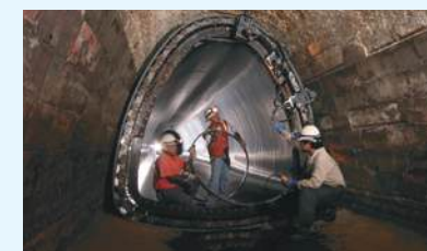
Pipe renewal construction in the United States
