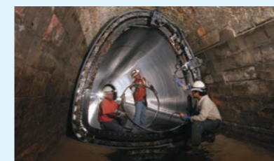
Pipe renewal construction in the United States
