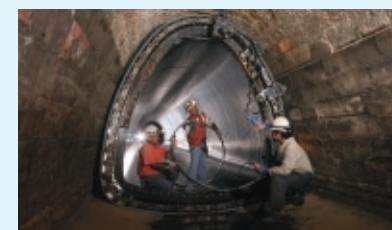
Pipe renewal construction the United States
