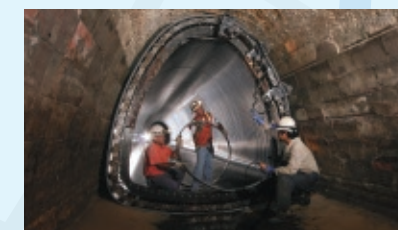
Pipe renewal construction the United States
