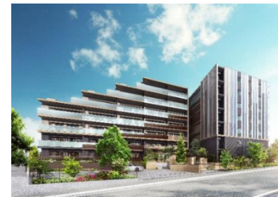
HEIM SUITE Nishi Chiba distinguished by its prominence in condominium development including Smart House and resilience, new normal, and design
