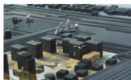
Rainwater storage tanks
