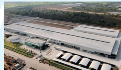
House production factory completed in 2013
