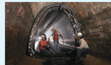
Pipe renewal construction in the United States
