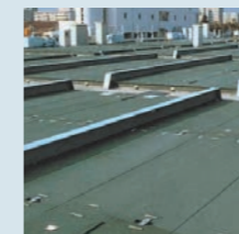
Cover lids for Sewage facilities (joint research with the Tokyo Metropolitan Government)
