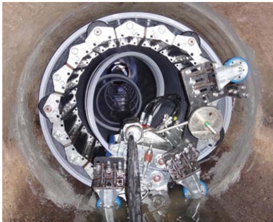
SPR sewerage pipeline rehabilitation method
