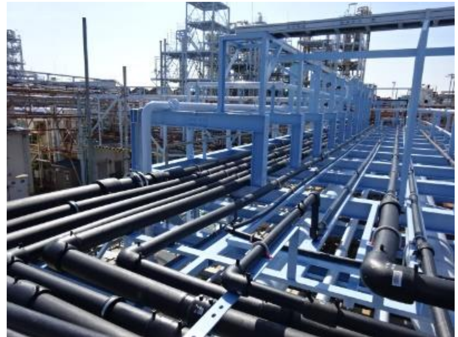
Earthquake-resistant high-performance polyethylene pipes
