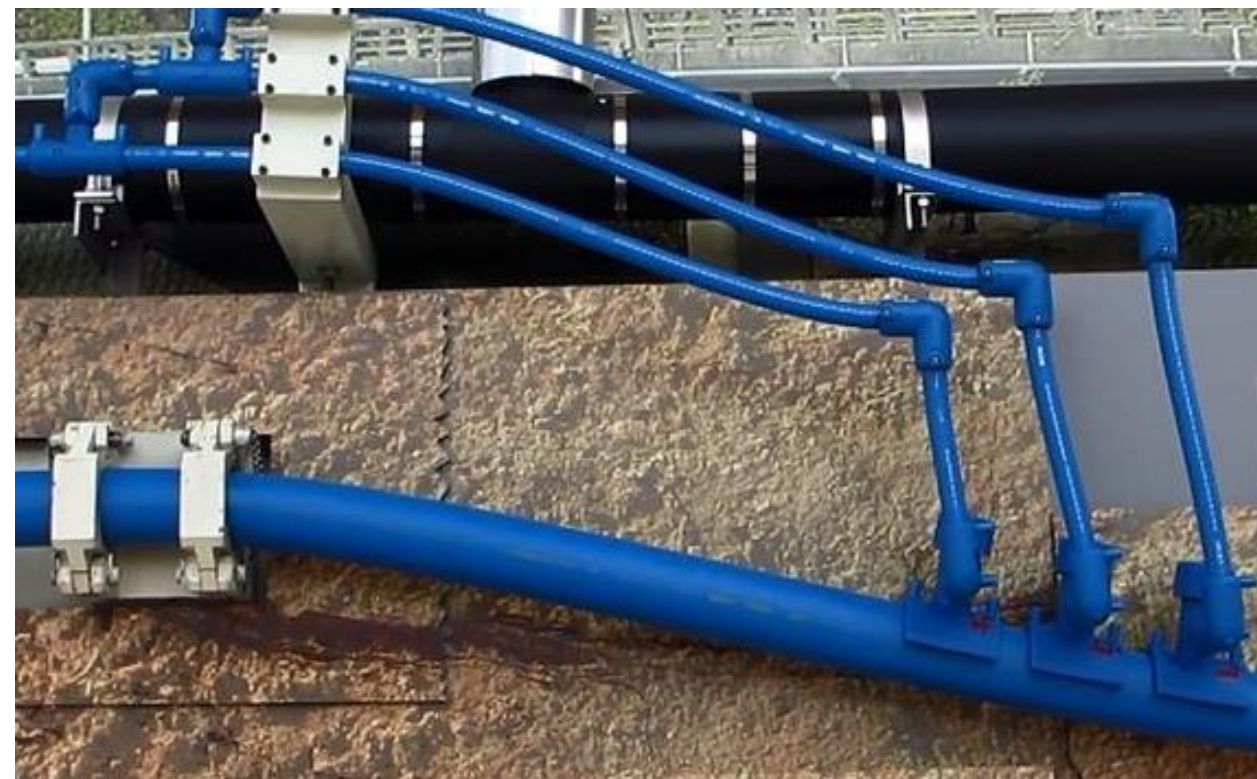
Earthquake-resistant high-performance polyethylene pipes
