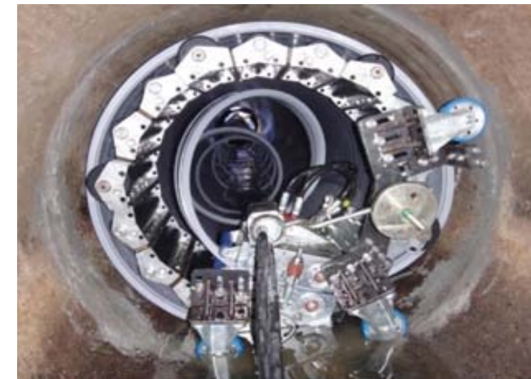
SPR sewerage pipeline rehabilitation method
