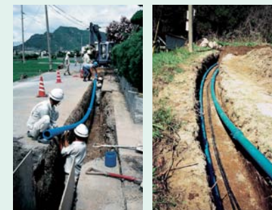
Laying high-function pipes with superior seismic capacity and ease of installation
