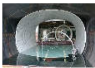
Rehabilitation method (New pipe making technology)
