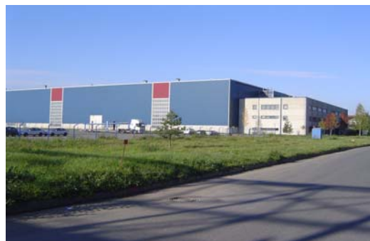
The plant site awaiting construction
