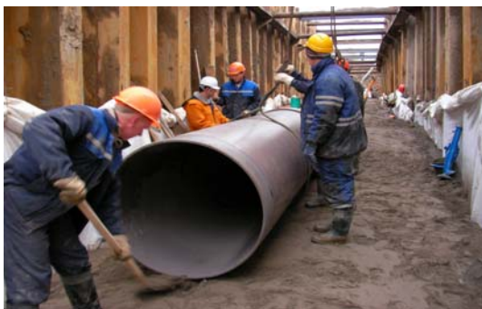
VKS employees work on an Eslon® RCP® pipes of \phi 1000mm
