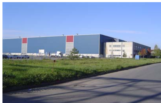
The plant site awaiting construction
