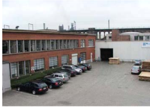
CPT Belgian plant (Liege, Belgium)
