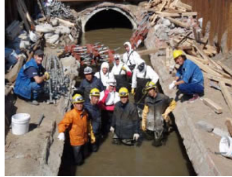
CPT personnel involved in Szczecin pipe-rehabilitation construction
