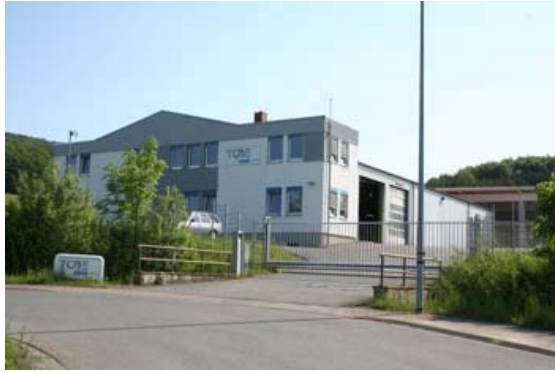
CPT headquarters/plant (Schieder, Germany)
