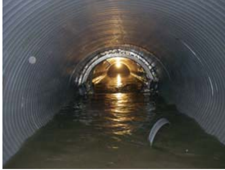
Interior of pipe under rehabilitation in Szczecin
