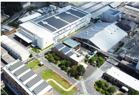
SEKISUI CHEMICAL CO., LTD. Shiga-Ritto Plant
