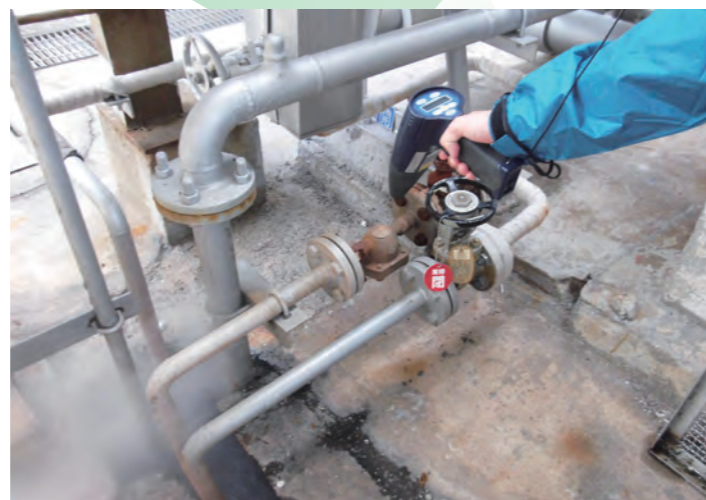
Inspection of heat leak condition of equipment at production site
