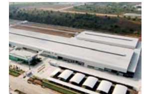
Factory for mass production of detached houses in Thailand
