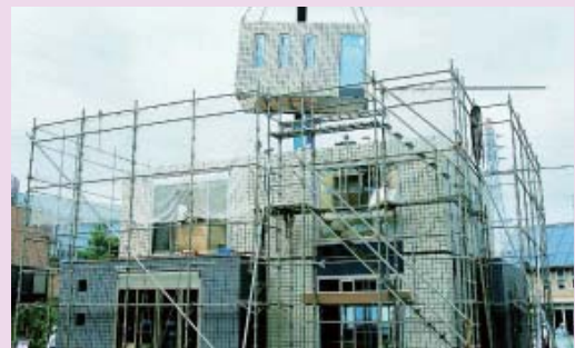
Swift on-site assembly completed in just one day
