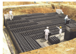
Rainwater storage systems contribute to torrential rain countermeasures
