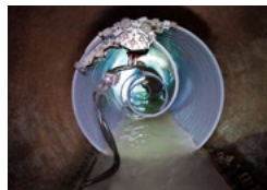
SPR Method contributes to aging infrastructure, including sewage pipes
