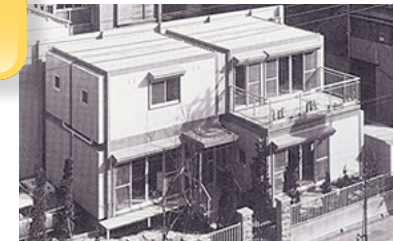
Unit construction method from 1971 SEKISUI HEIM goes on sale (world first)
