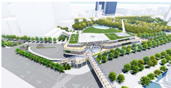
Scheduled for installation at the Umekita (Osaka) Station plaza area when it fully opens in 2025 * Subject to change in the future by agreement between the related parties. Image provided by West Japan Railway Company
