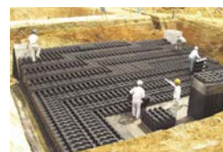
Rainwater storage systems contribute to torrential rain countermeasures
