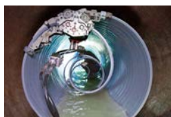
SPR Method contributes to aging infrastructure, including sewage pipes
