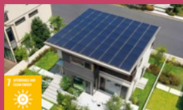
A large capacity solar power generation system
