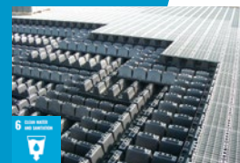
Rainwater storage system
