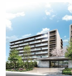
HEIM SUITE ASAKA condominium
