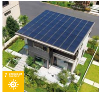
A large-capacity solar power generation system
