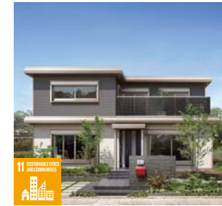
External walls (Eco-chante) renovation
