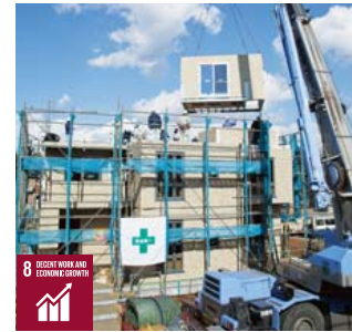
A housing unit being installed
