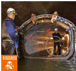
9 INDUSTRY, BARRIERS AND INFRASTRUCTURE Sewage (Spirally) Pipe Renewal (SPR) Method
