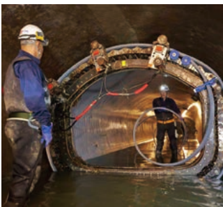
Sewage pipe rehabilitation
