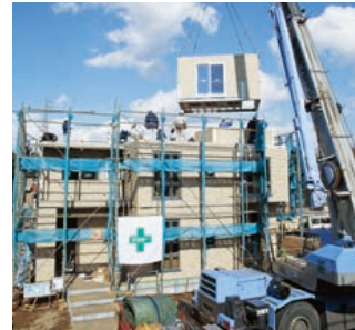
A housing unit being installed
