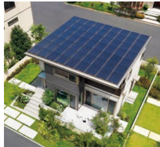
A large-capacity solar power generation system
